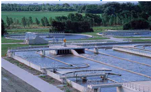
(9) Biological wastewater treatment, Carrousel Geestmerambacht (Source: DHV) [for high resolution version, see CD-rom]
